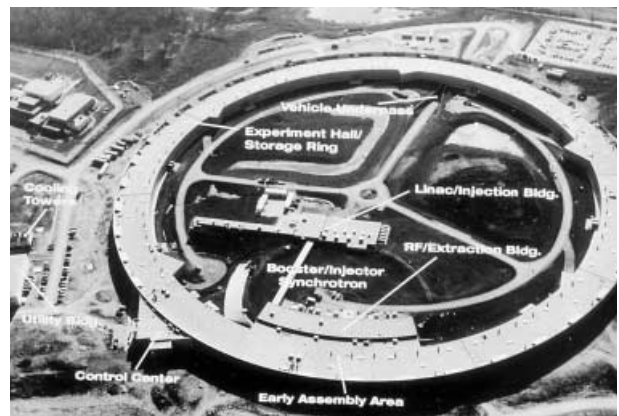
Fig. 18. Advanced Photon Source (APS), Argonne Laboratory, USA. Scale of the machine can be judged from automobiles and tractor-trailers on left-hand side of photographs.
